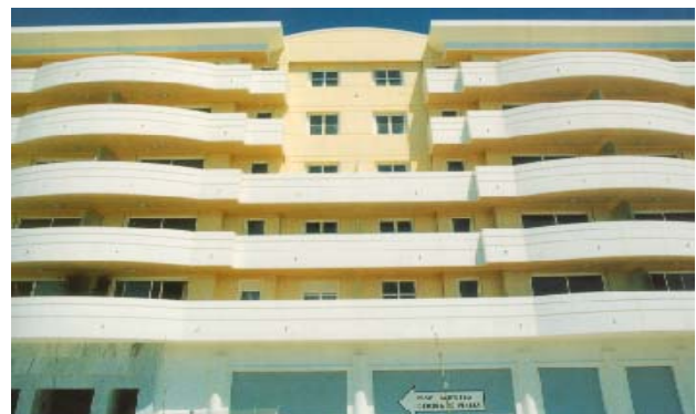
Figure 2: Aspect of Typical GRC Facade
