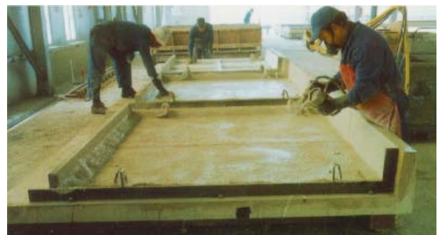
Figure 5. Manual spraying and compacting operations
