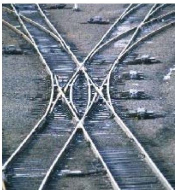
Figure 1: Example of Railway Switch Point Assembly
